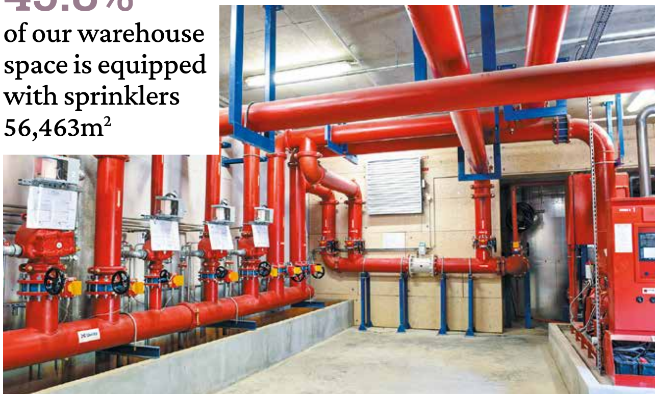
Sprinkler system at Sferaco
