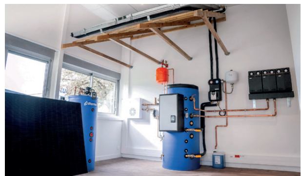
Installation of a solar water heater at Thermador
