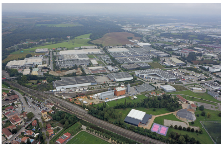
View of the Saint-Quentin-Fallavier business park
